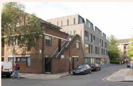
Kensington Day Centre (front)
